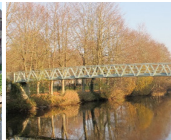
La passerelle. Photo © ASP
